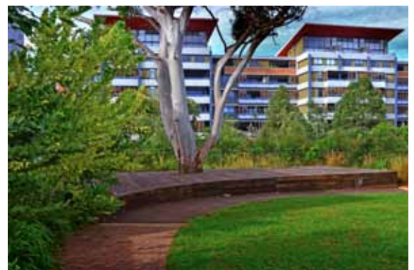
Timber decking isolates contaminated soils whilst protecting trees.
