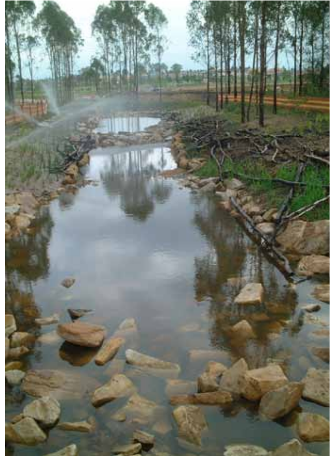
Newly constructed creekline complete with habitat logs
